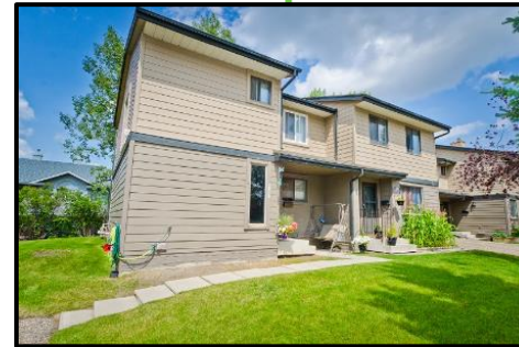
Beddington Heights Village (Calgary) Q2 2024 62 Suites $269k per suite Est. 4.25% - 4.50% Cap Rate
